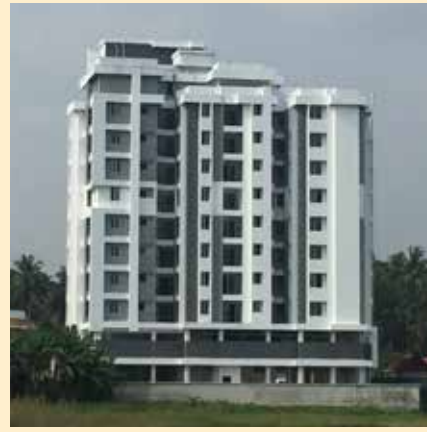
OPAL Kuttumukku, Thrissur
