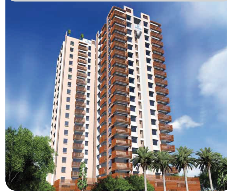
HERITAGE | Punkunnam, Thrissur Ongoing Project
